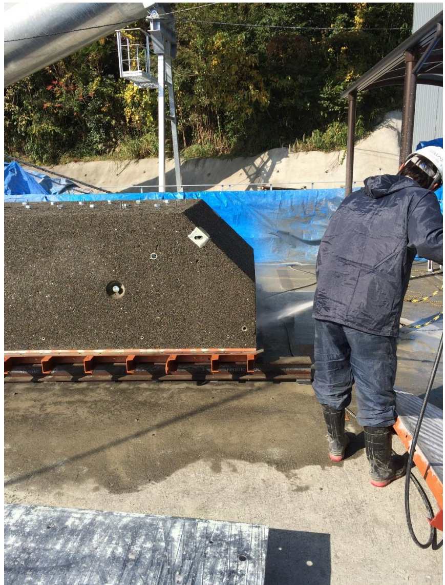
1Wash-out with high-pressure spray equipment
